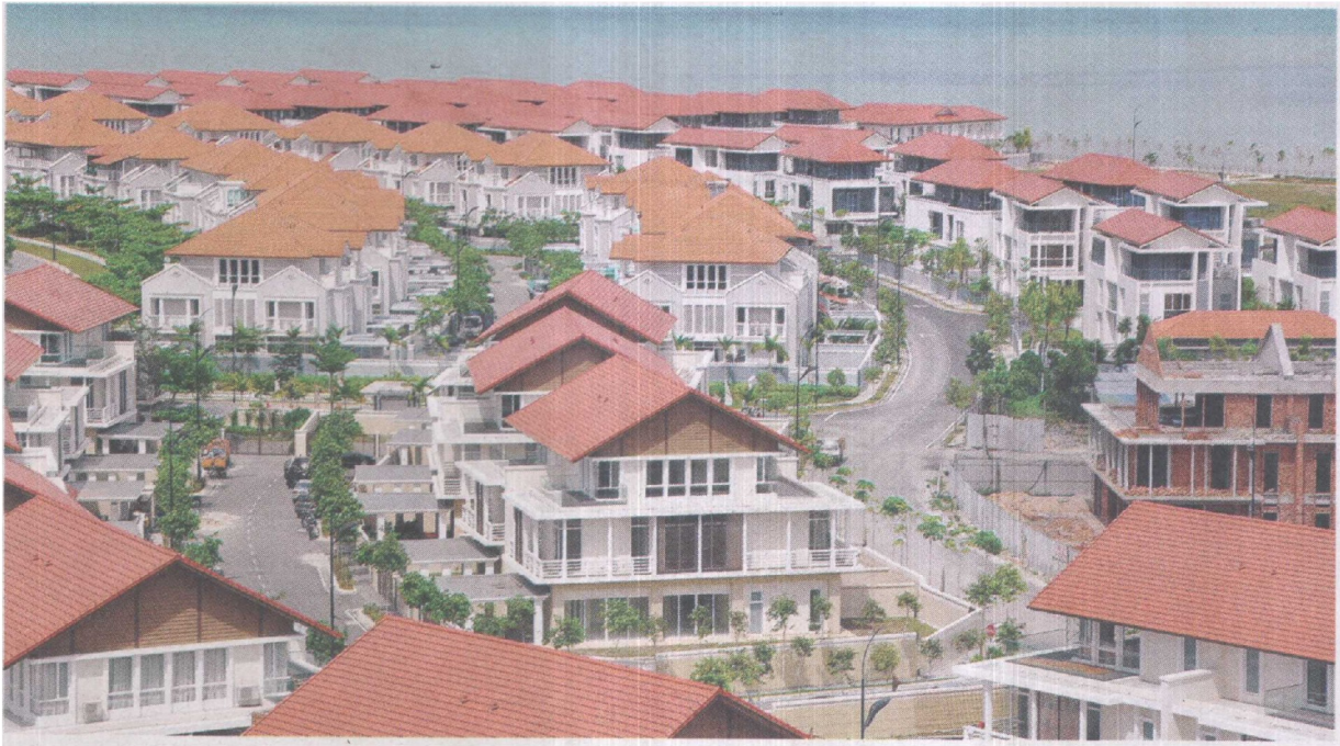
Heat absorbers: Concrete surfaces absorb heat, causing the heat island effect. If roofs and buildings are painted white, they will reflect the heat instead.
