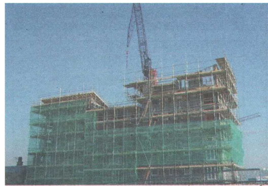
Multi-storey timber frame structures used on construction sites.
