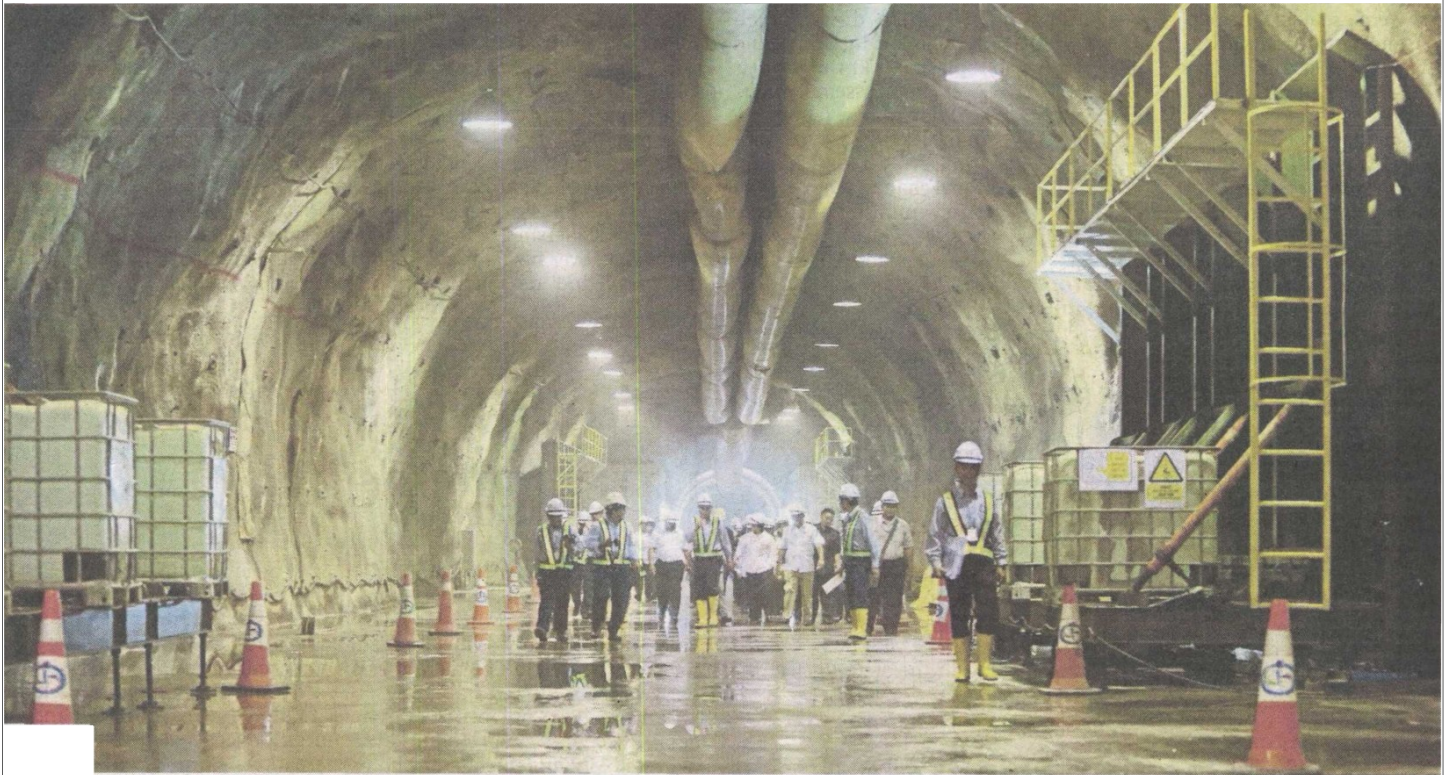
Workers at the Pahang-Selangor Raw Water Transfer Tunnel . File pic
