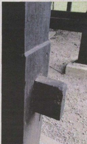
The posts of the house are secured using tenons and mortises, and the legs are each placed on a stone slab.
