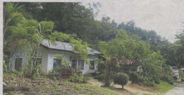
Some houses in Kampung Orang Asli Bukit Lagong are located very close to the proposed site.
