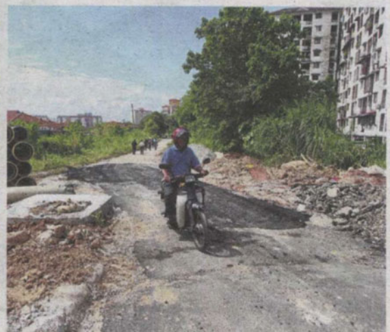
Very few motorists use Jalan Besar Kepong as the roads are in bad shape.
