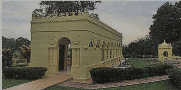
The Makam Sultan Abdul Samad at the Royal Mausoleum in Bukit Jugra was constructed according to Moorish and Islamic architecture
